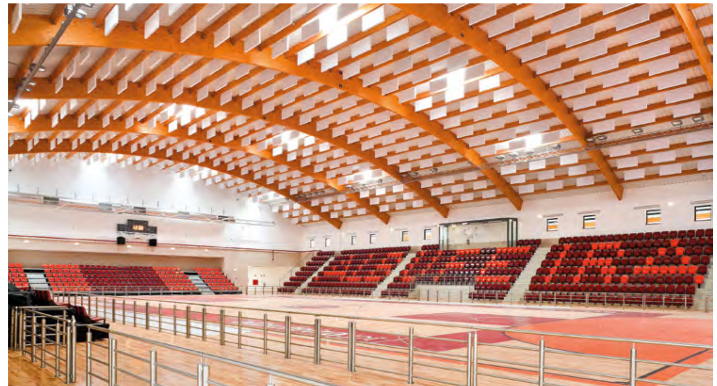
PAVILHÃO GIMNODESPORTIVO SPORTS PAVILION ALBUFEIRA
